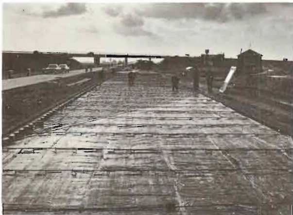
Left: Laying the 9 mm diameter wires for post-tensioning by the Strabed-H.B.M. system
