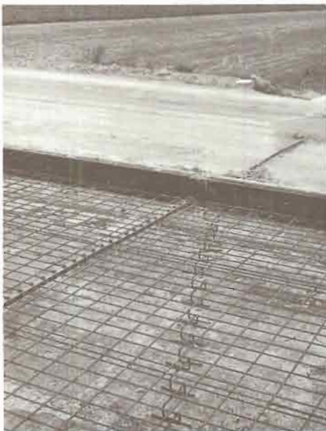
Figure 55. Lateral support of tendons in a horizontal curve. (See also Figure 44.)
