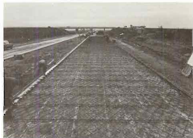
Left: Laying the 9 mm diameter wires for post-tensioning by the Strabed-H.B.M. system
