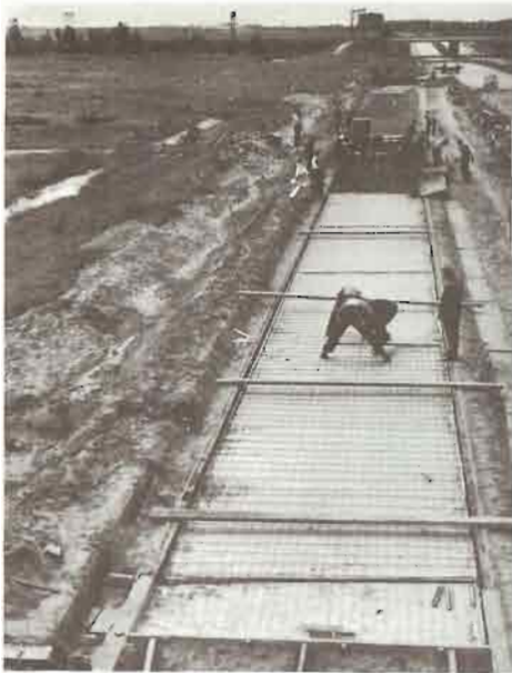
Figure 29. Concreting the experimental slab at Leidschendam
