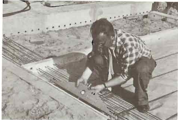
Figure 34. Device for measuring tension in wires
