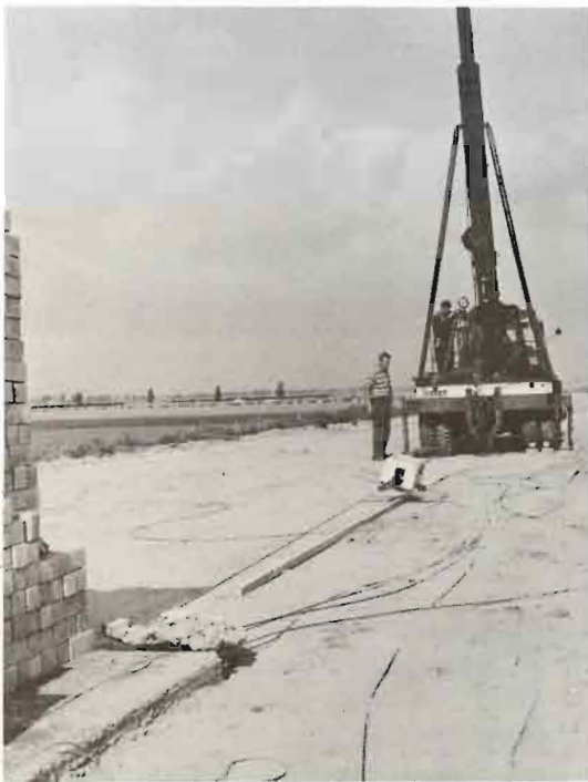
Figure 51. Tensioning a tendon with the aid of a pulley-block mounted on a lorry
