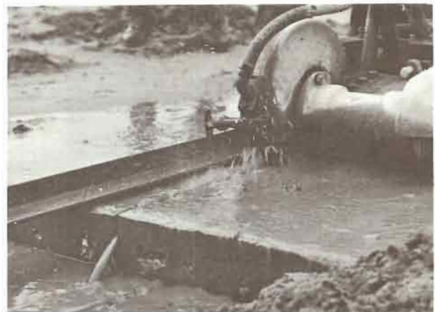
Figure 56. Sawing the concrete and the tendons at a joint
