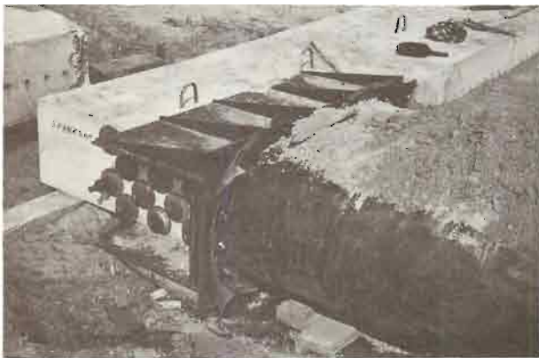
Figure 31. Detail of pre-tensioning frame
